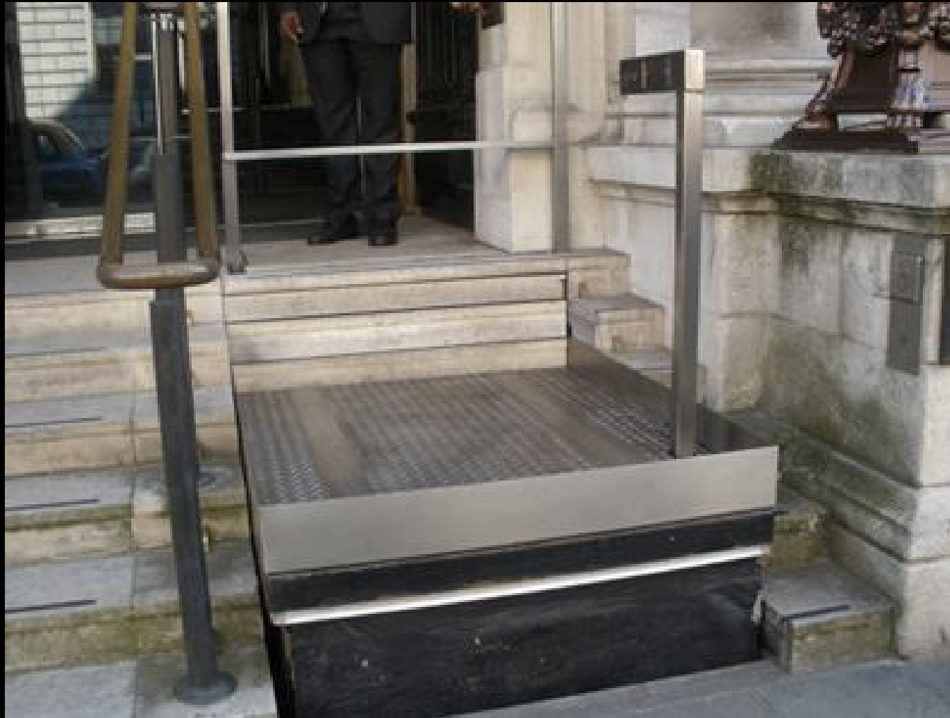
London, Institution of Civil Engineers
